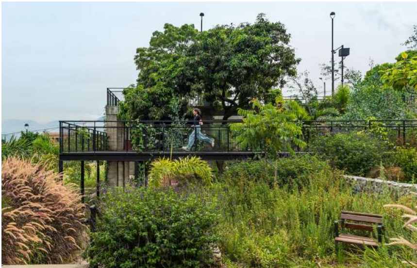
Lush greening surrounds the site's structure and welcomes activity at different levels (Connatural)
