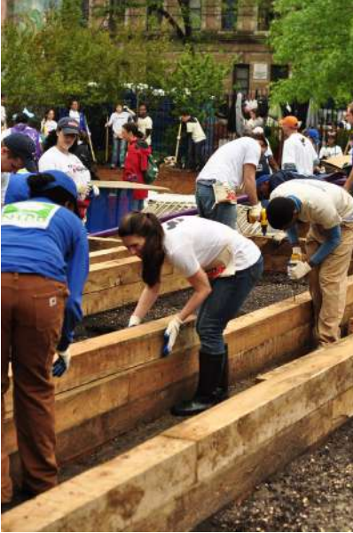
Volunteers working together to build the project (SCAPE)
