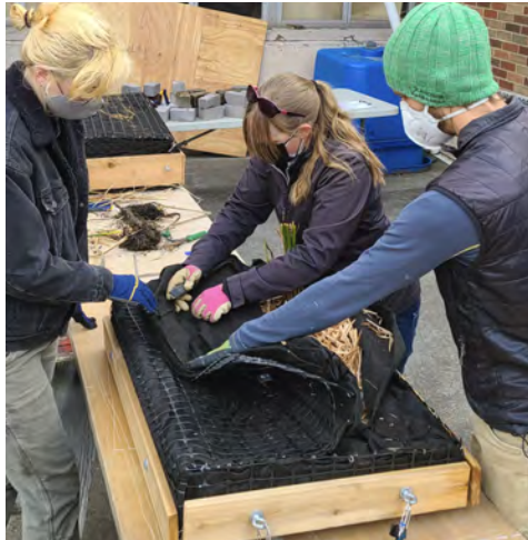
Figure 6.1: UW students assisting Jenn Engelke in constructing prototypes for the floating wetlands.
