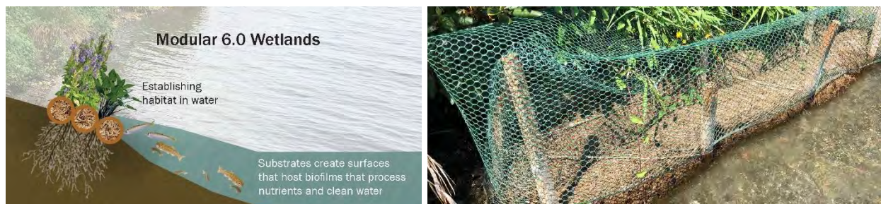
Figure 4.2: Modular 6.0 wetlands made from coir logs as a living shoreline extension
