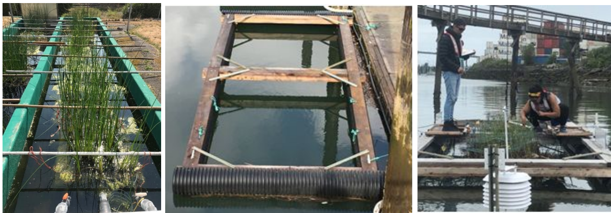
FIGURE 3a. Biofilter construction at UW hatchery (left), BioBarge construction at T-102 (middle), and deployment at T-108 (right)
