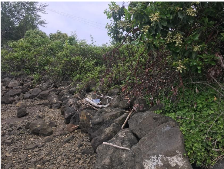
Figure 5. Vegetated riprap shoreline placement at T-108.
