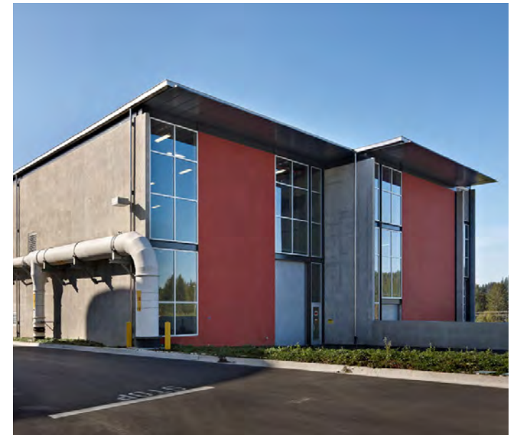
Figure 50: Brightwater Treatment Plant (Case Study - p. 64)
