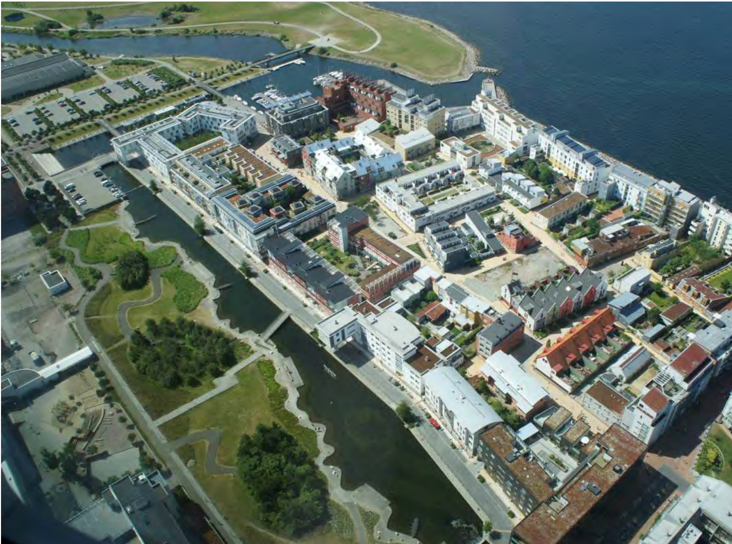
Figure 76: Western Harbor Aerial View
