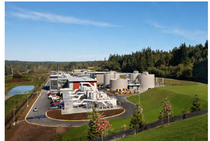
Figure 61: Brightwater Treatment Plant, , Mithun Architects of Seattle.
