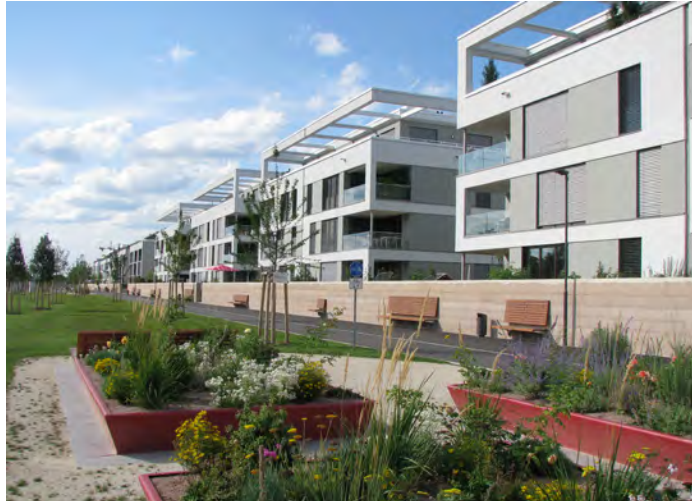
Figure 57: Bahnstadt Urban Village, Germany
