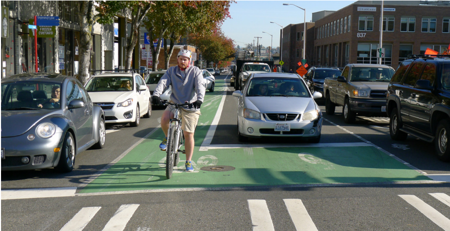
A Bike Box gives bicyclists a place to wait at the light while providing protection from right turning vehicles. In Copenhagen bike boxes are often combined with bicycle lights that change several seconds before the vehicle light allowing them to move from in front of cars.
