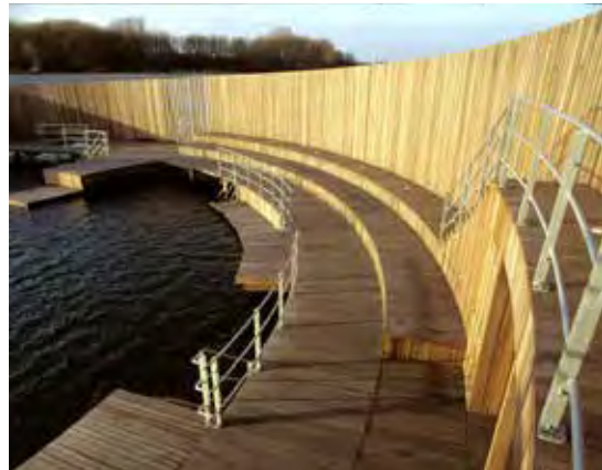
Platforms on multiple levels
