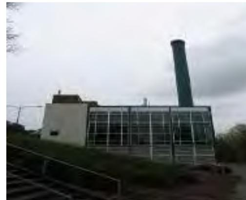
With 8 miles of underground tunnels, the UW Power Plant is the main generator of campus wide energy. Providing 174 campus buildings, including the Medical Center, with steam, chilled water for air conditioning and compressed air, the Power plant is a proven energy asset. In one hour, 800,000 pounds of steam, 12,000 tons of cooling and a the capacity to provide emergency power within 10 seconds of an outage.
