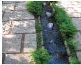
Stormwater from Roof
