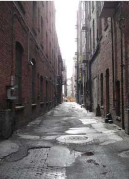
Typical Alley Condition Source: William Payne
