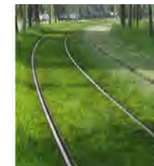
Bioswale Streetcar Alignment as Runoff Filter
