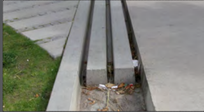
[gutter infill for crossing]
