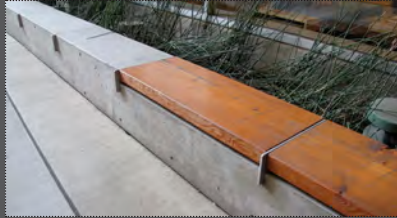
[wood inset on poured in place concrete benches]
