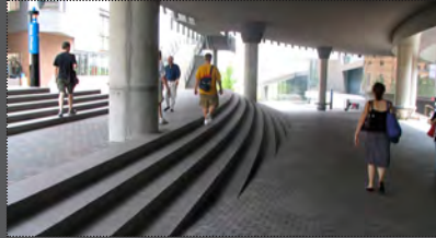
[stairs merging into sloped pathway]
