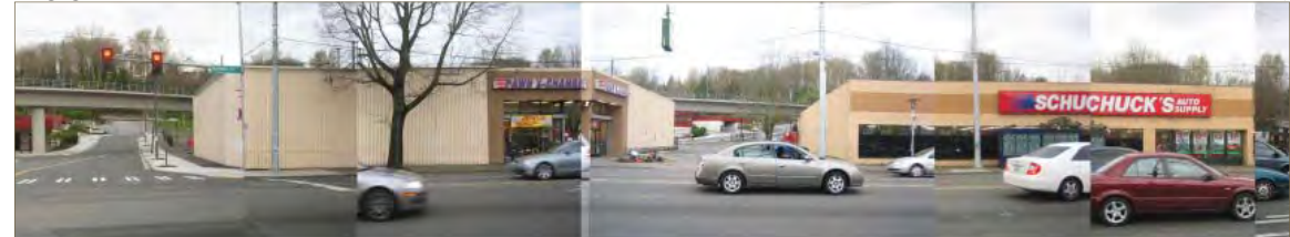
Existing View of Site From Rainier Ave.
