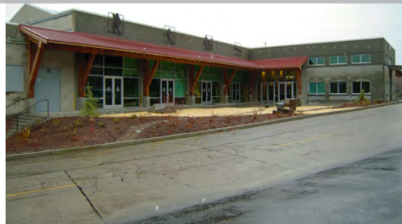
Mountaineers Club Seattle, USA source: Clark Design
