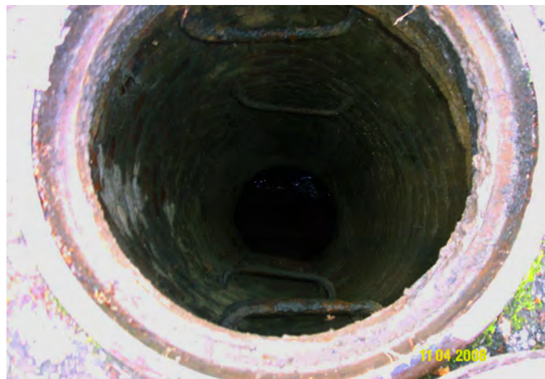
view into stormwater pipe source: GGLO
