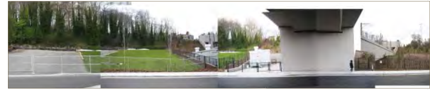
Existing View of Site Under Light Rail Structure
