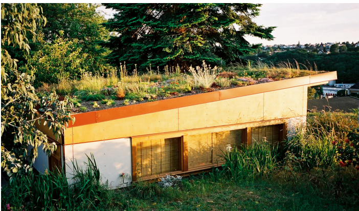
Private garage roof. Photo: Rob Harrison (designer & owner).
