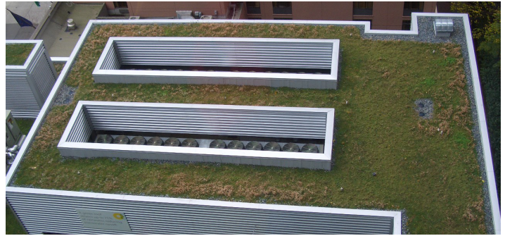
The Hyatt at Olive 8 green roof. Photo: Annika McIntosh, 2009.
