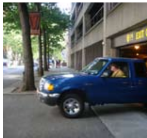
Asphalt communicates car space, so even though the sidewalk level remains consistent, the design tends to prioritize cars driving in and out of garages.
