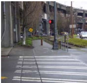
The shared walking and bike path along Alaskan Way has numerous crossing lights. A bicycle route located on the waterfront side would create a less interrupted path and provide views for users.
