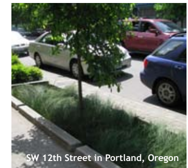
Street-side filtration cells are a simple and unobtrusive way to add green to the streets.
