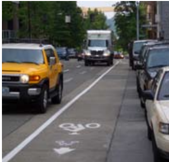
A “bike lane” is marked by a solid line. It is placed between parked cars and driving cars causing cars to drive across or open doors into the bike lane. This requires drivers and passengers to respect the bike lane so as not to open the car door and hit a cyclist.
