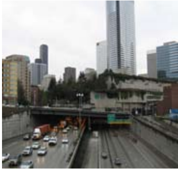
I-5 creates a big scar in the city. It is very difficult, if not impossible, to create a high quality city fabric next to a large freeway.
