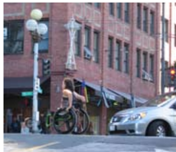
ADA ramps are crucial for people with disabilities, but they ought to be placed in line with the crossing and not in the corner.
