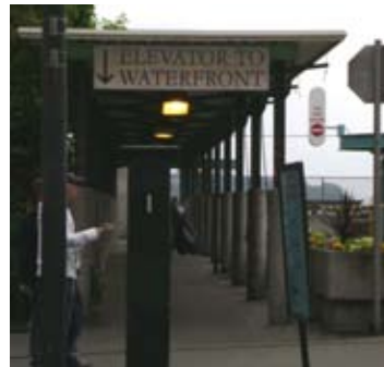
It's important that elevators are safe, visible, and clean so people feel welcome and safe. The present elevators have room for improvement.
