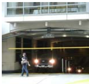
The bar across the garage exit increases safety if it forces cars to fully stop before driving across the sidewalk. It can also alert drivers to be more aware of pedestrians crossing the exit.
