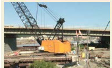
June 3, 2013 construction photo [King County Department of Transportation]
