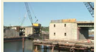
June 3, 2013 construction photo [King County Department of Transportation]
