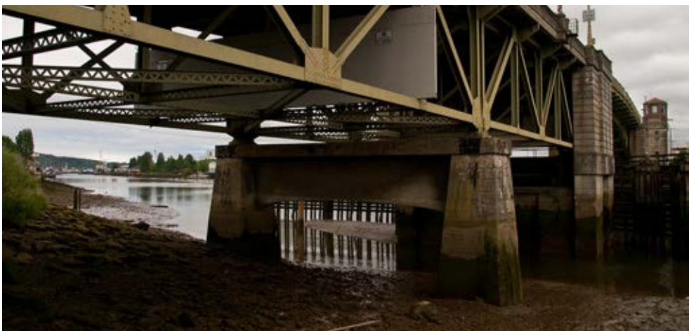
Existing South Park Bridge Conditions
