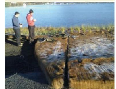
The wetland was constructed from over 400,000 plastic bottles (imported from the U.S.) topped with coconut fiber matting and over 20,000 native plants. Modules were bolted together with steel and wire (like knitting a scarf row by row).
