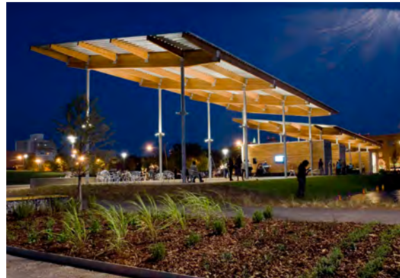
The pavilion welcomes people to the park, providing shade, cover, and light at night (Tom Leader Studio)
