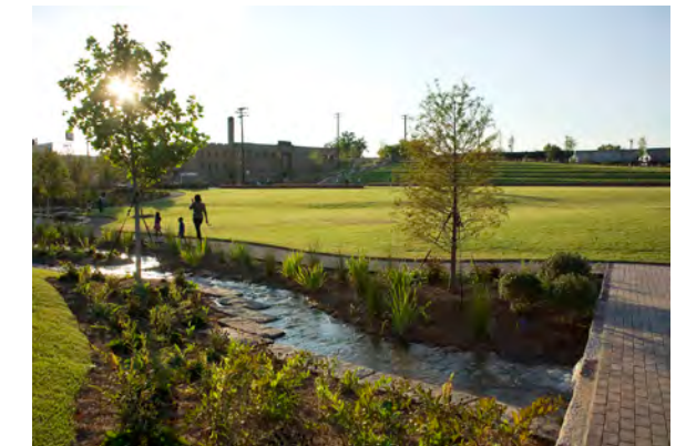
Stormwater is circulated through water bodies on site, using plants for biofiltration (Tom Leader Studio)
