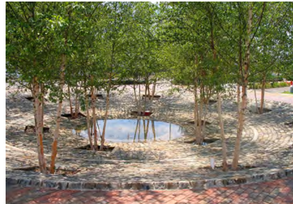
"Birch Bowl" is a stormwater retention pond and play feature (Tom Leader Studio)
