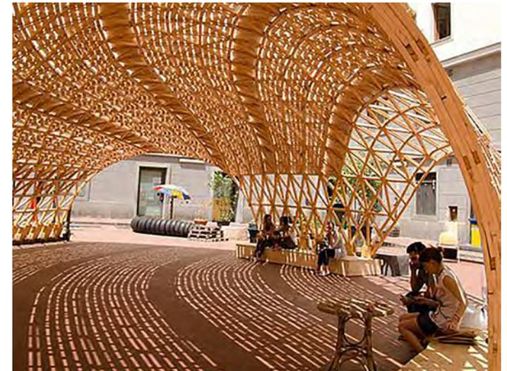
Figure 63: Cafe with a gridshell structure
