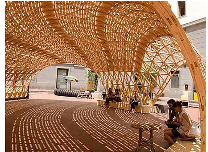
Figure 63: Cafe with a gridshell structure
