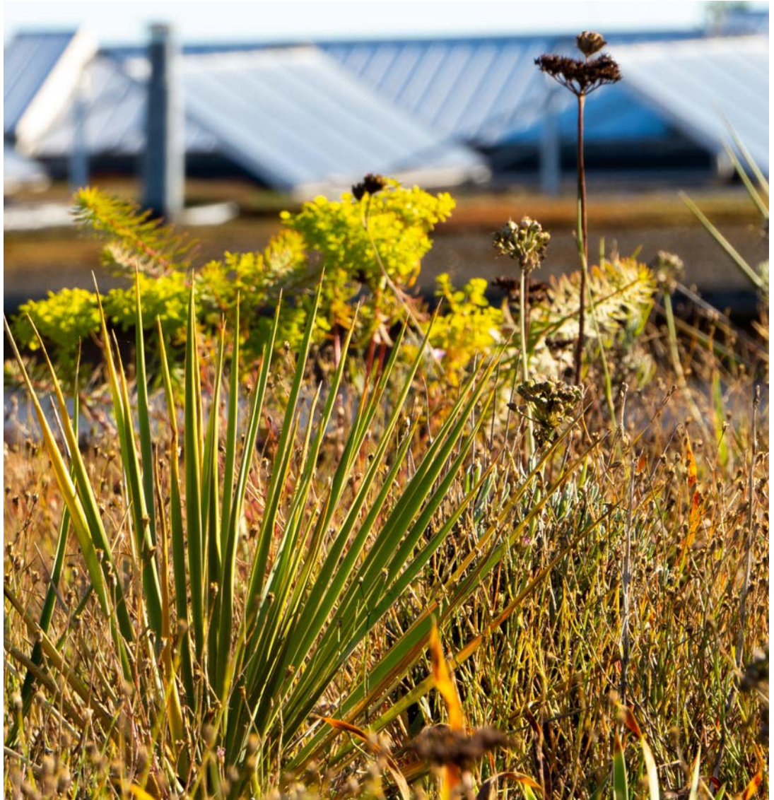
Biodiverse rooftop “rock” garden. Constructed with cellular glass, sand, pumice, and biochar substrate with a range of unique plants adapted to difficult environments. Solar panel roof garden in background. Created by Peter Korn; hosted by the Scandinavian Green Roof Institute in Malmö, Sweden.
