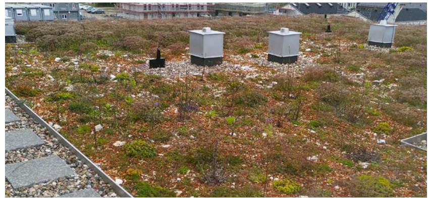
Second year of growth: a lush biochar amended area can be seen in the background with an intentionally harsh limestone steppe area in the foreground. 1
