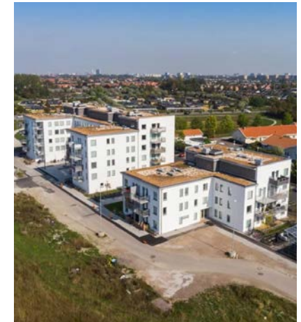
Buildings with limestone steppe roofs. 4
