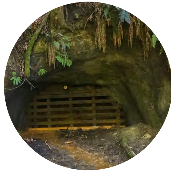
6. Evidence of a coal mine found at 15 mile creek. These mine entrances are dangerous and sealed shut.
