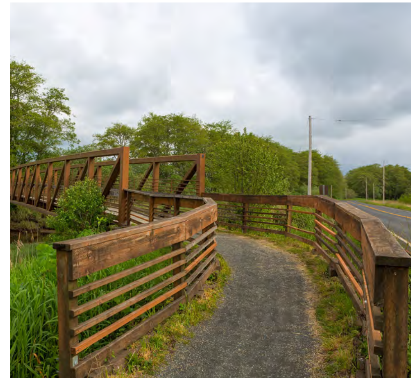
Example of an unpaved ADA trail in a natural area..Image from Adobe Stock
