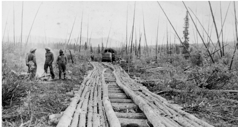
Historical photos such as this one of a corduroy logging road could be used on interpretive signage. Image from Timberlake Collection, UW Libraries
