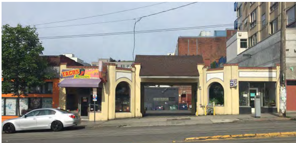
This block face has a variety of functions and use of materials. Quality and maintenance of materials vary, leading to a somewhere in-between score.
