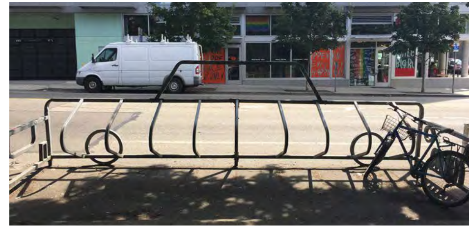
A large on-street cluster bike rack on 12th Avenue minimizes disruption to pedestrian walking flow.
