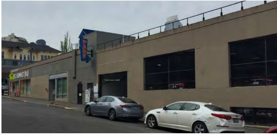
A parking lot with an unengaging facade dominates the block.
