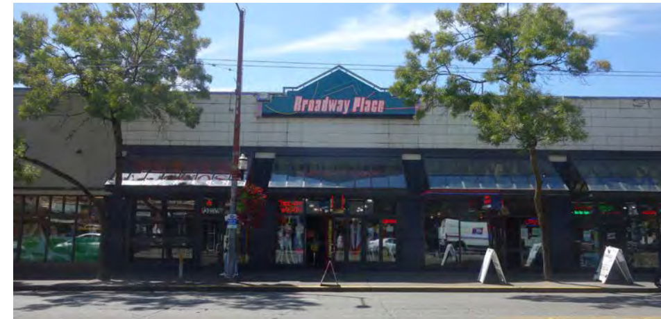
This building has small units, a variety of functions, and consistent awning coverage that establishes human scale and aesthetic continuity between businesses.
