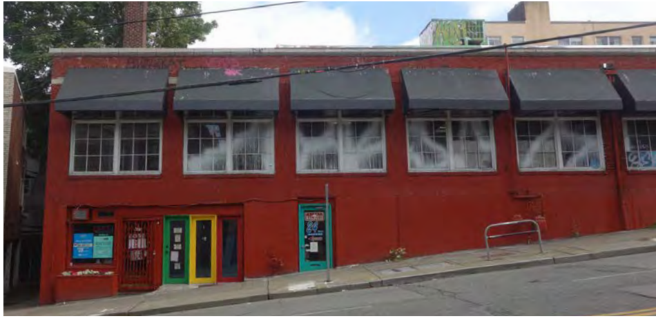
This frontage on the steep slope of Denny has ground floor retail but only modest activation. Awnings are not at eye level. Seating options are lacking.
